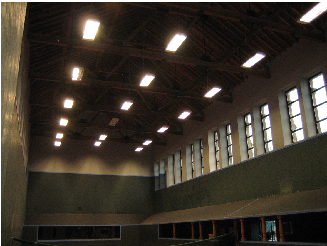
Another view of the new lighting—there are 27 light units (2 are not needed and therefore are spare but can be switched on if necessary).
